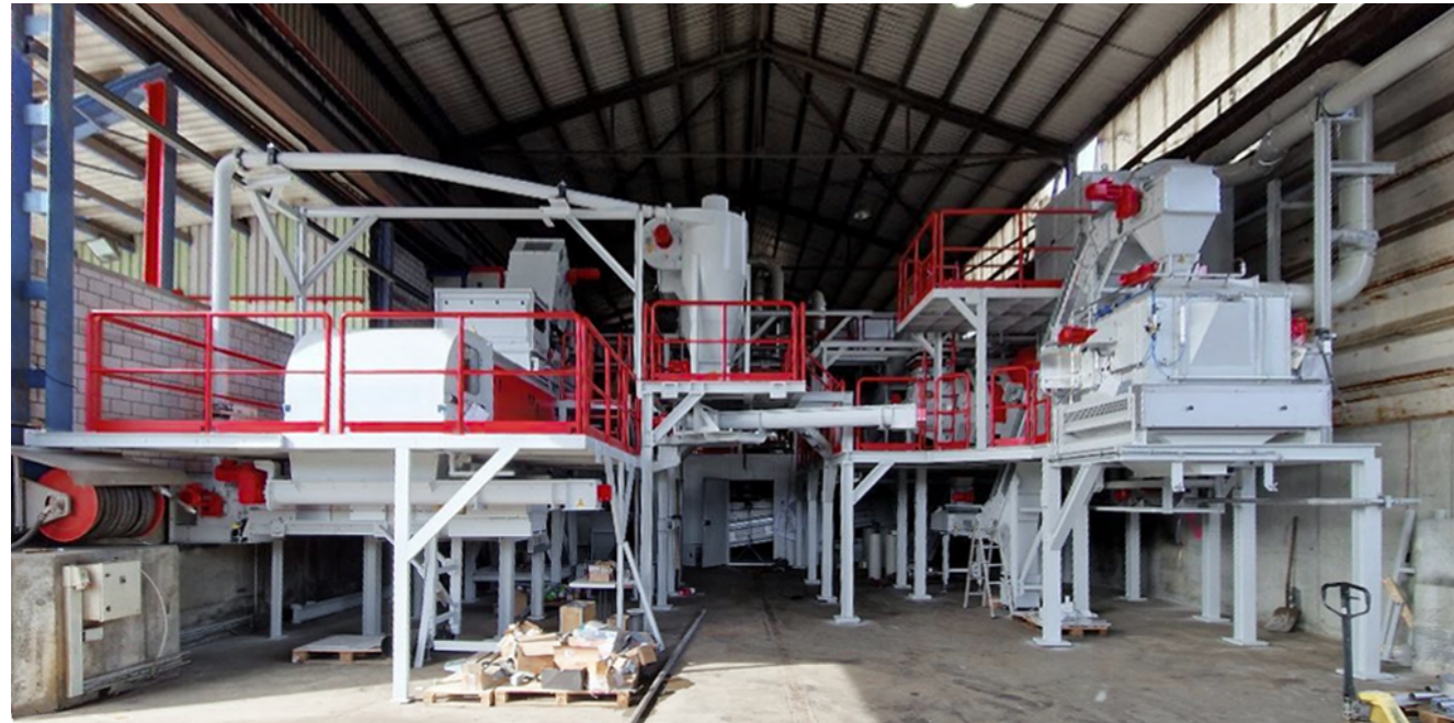
E. Flückiger AG refrigerator recycling plant from URT under construction. Left: eddy current separator, right: pellet cooler.
