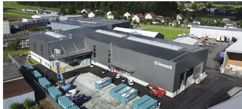
New production site of Immark AG Aarwangen BE.
