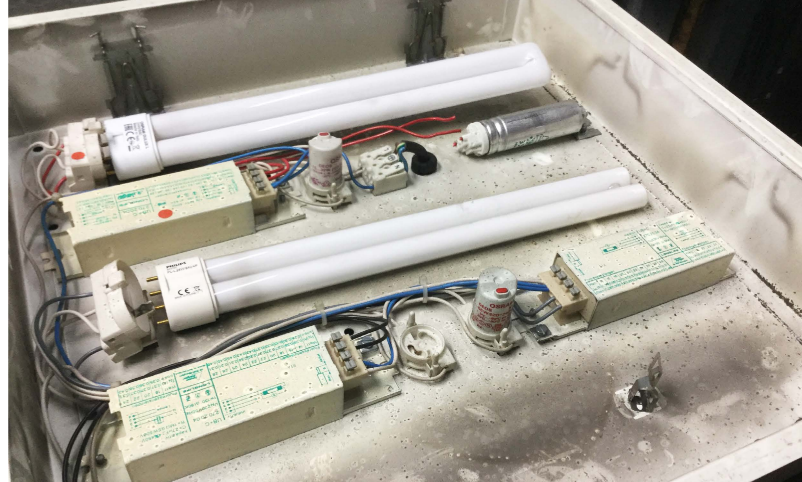
Photo 1: In this square lamp, the ballast unit consists of three inductive parts and a capacitor.
